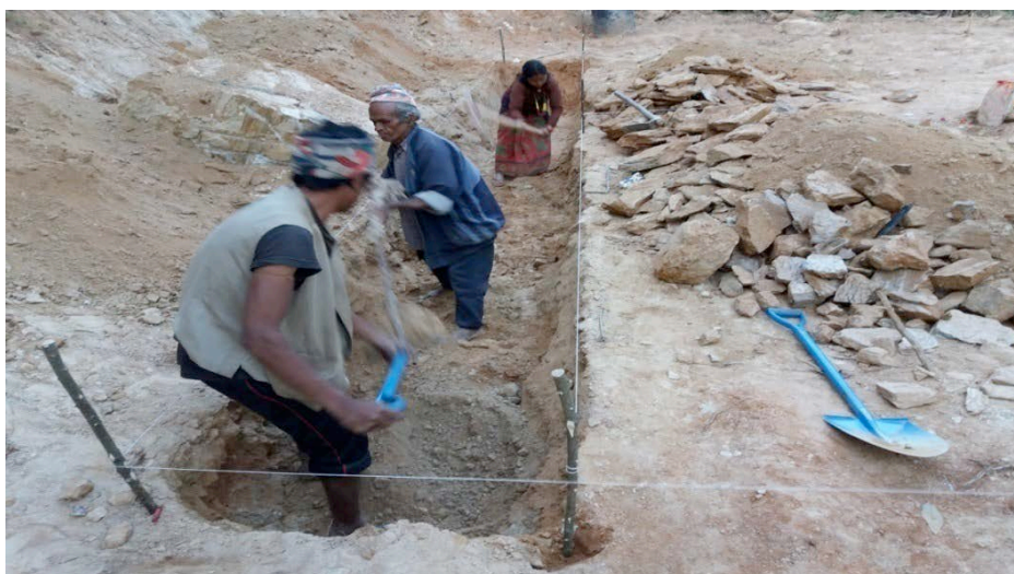
Figure 4 (Workers digging hole for foundation of CRC building Namdu, Dolakha)
